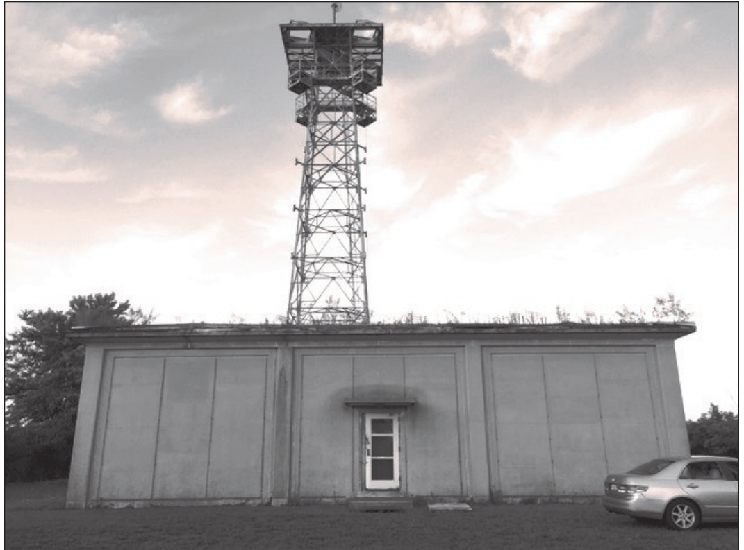
View of the building and tower at the former AT&T Long Lines Shandon site. The tower is 120 feet tall to the top work platform and the building measures 55 by 55 feet. The beacon is located on the left side of the tower in this view, on the top platform.
